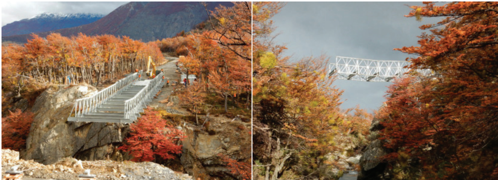
Launching of a panel bridge
