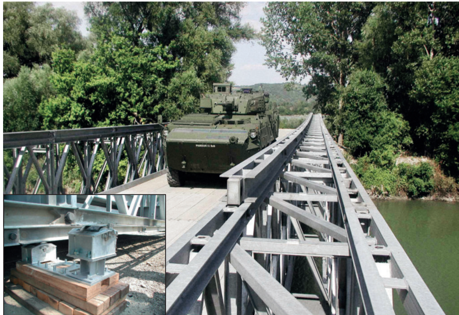
The panel bridge in Klosterneuburg near Vienna was built jointly with the Austrian Federal Armed Forces.
